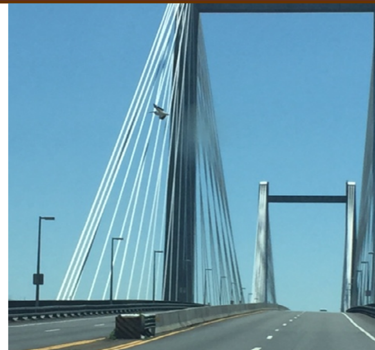
Ed Hendler Bridge, Kennewick, WA
